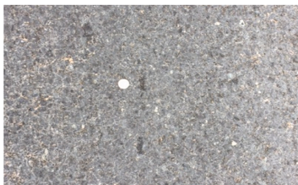
a) Al Jemaiya street (1 year with NMAS of 12.5 mm with MTD of 0.65 )
