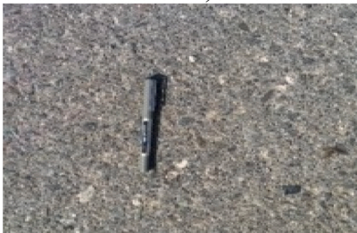
c) Dukhan highway (6 years with NMAS of 19 mm with MTD of 0.88 )
