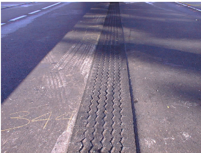
Fig. 4. Photo of Section 7C (bi-directional loading with no wander).
