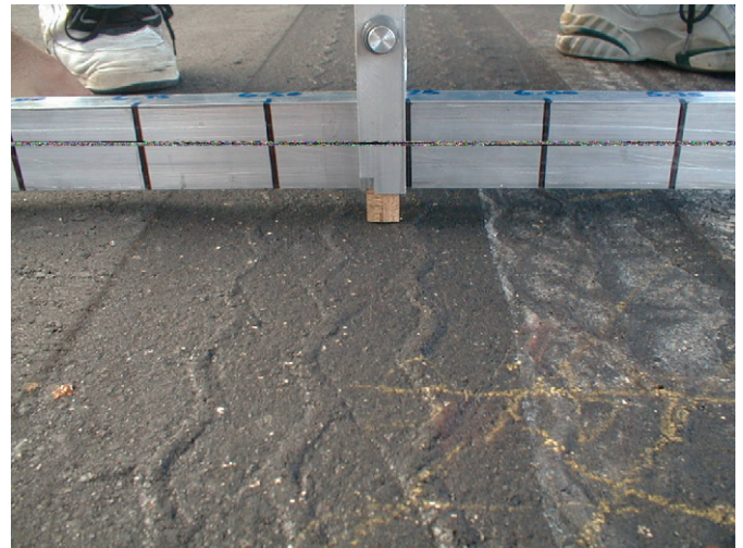
Fig. 2. Photo of straight edge used for measuring rut depth.
